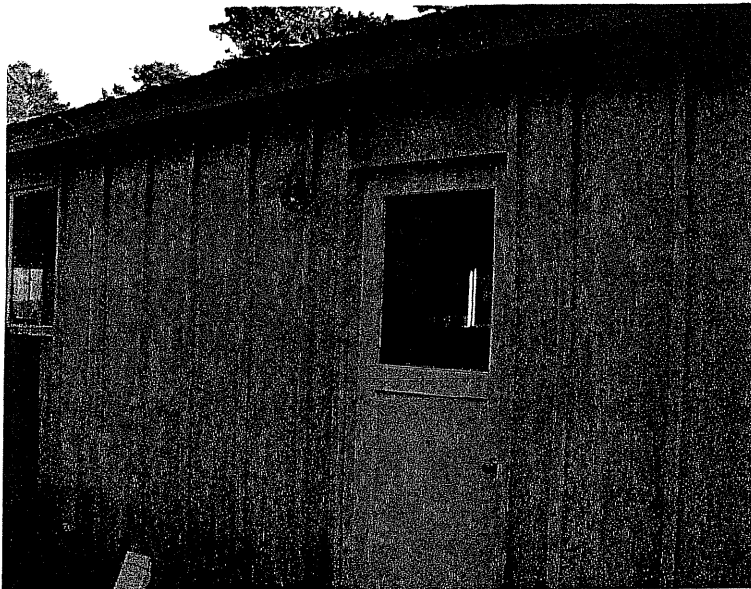
View of North Side of Garage
