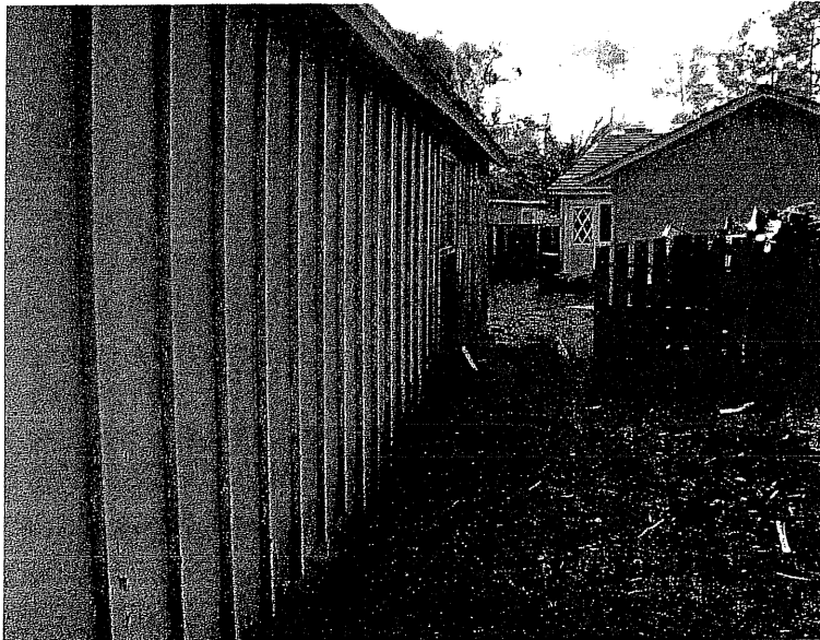
View of North Side of Garage
