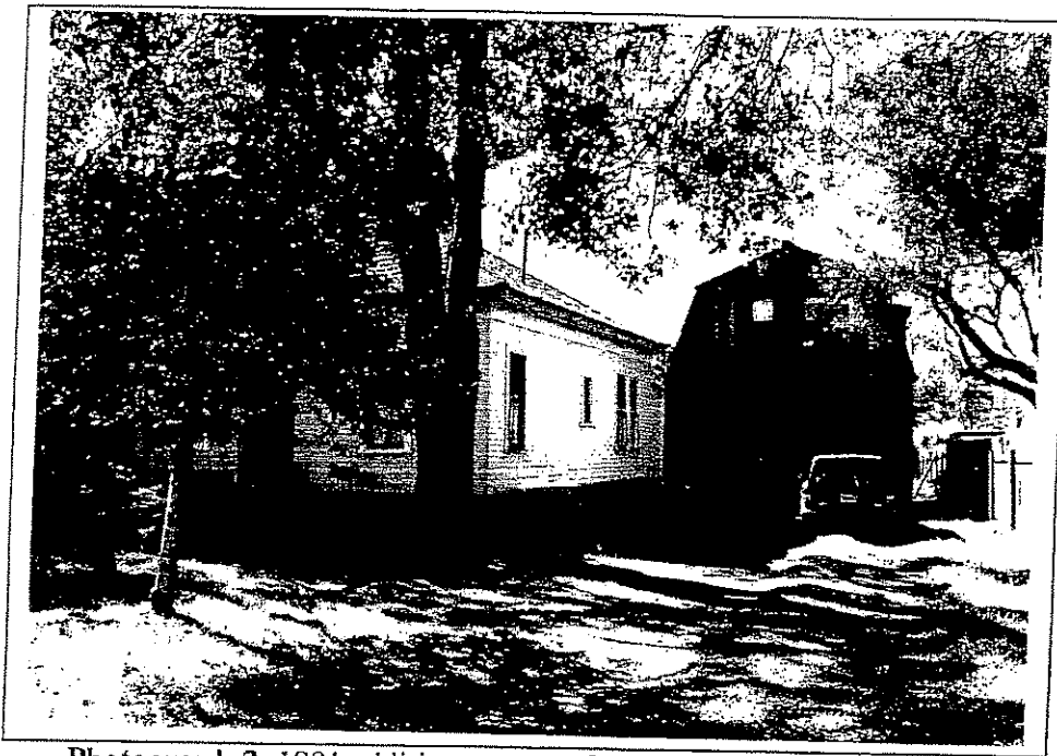
Photograph 2. 1981 addition, camera facing west, March 14, 2002.
