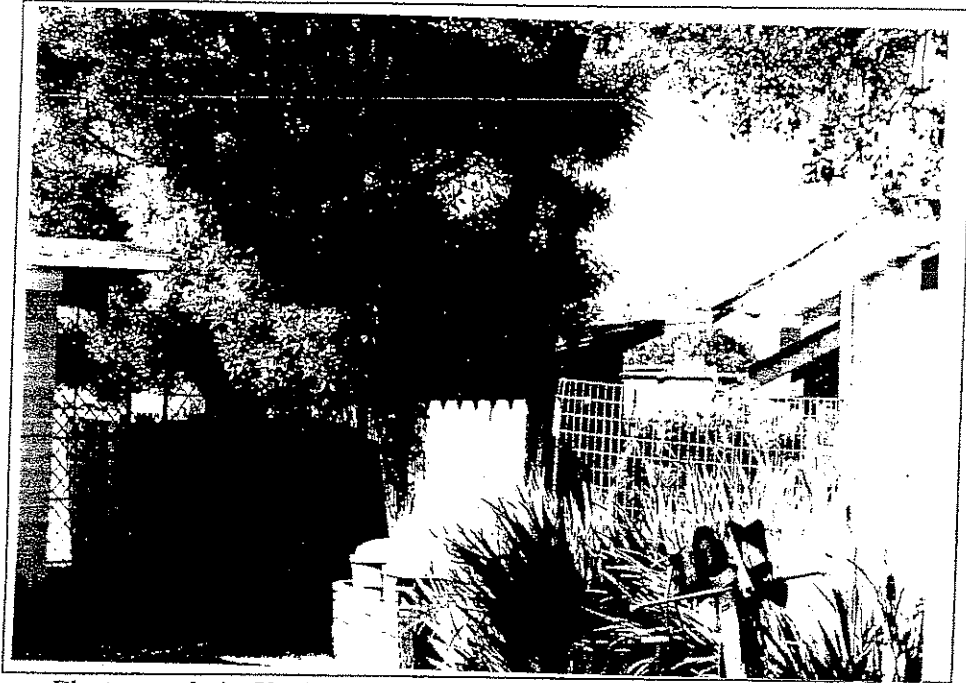
Photograph 4. Sheds (at right), camera facing west, March 14, 2002.
