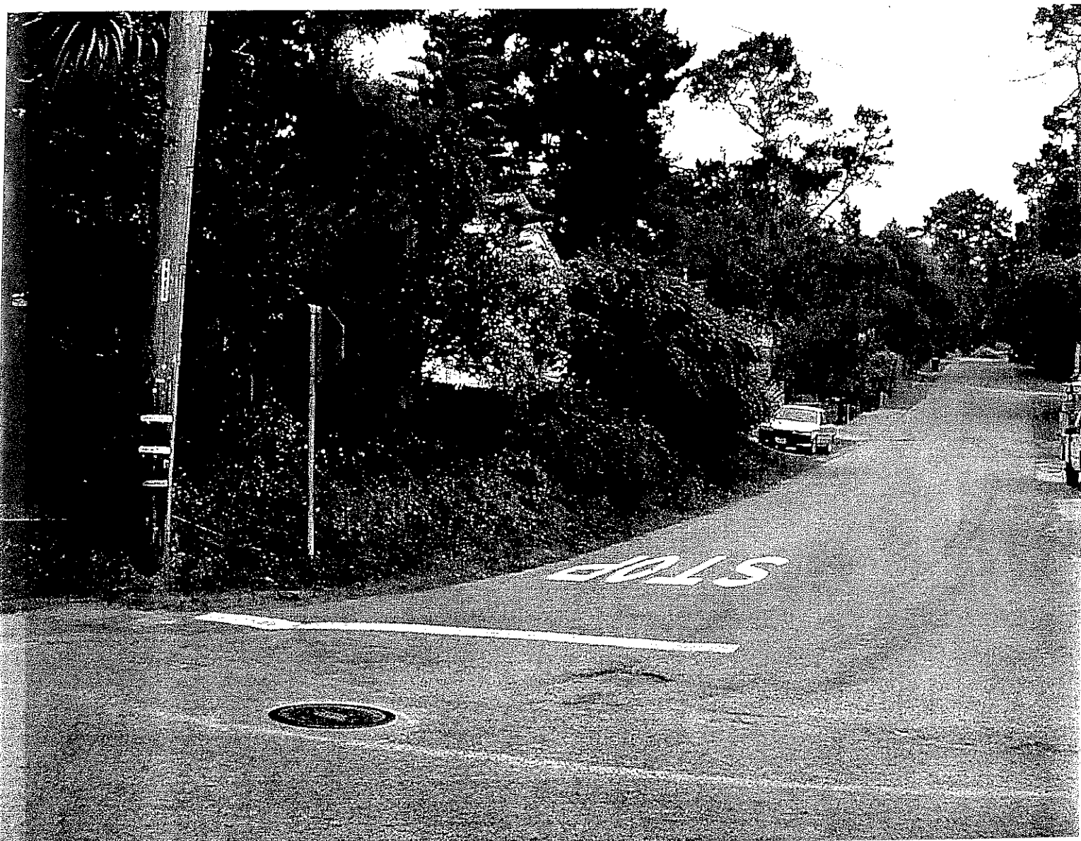
1129 DAVID AVE (VIEW FROM INTERSECTION)
